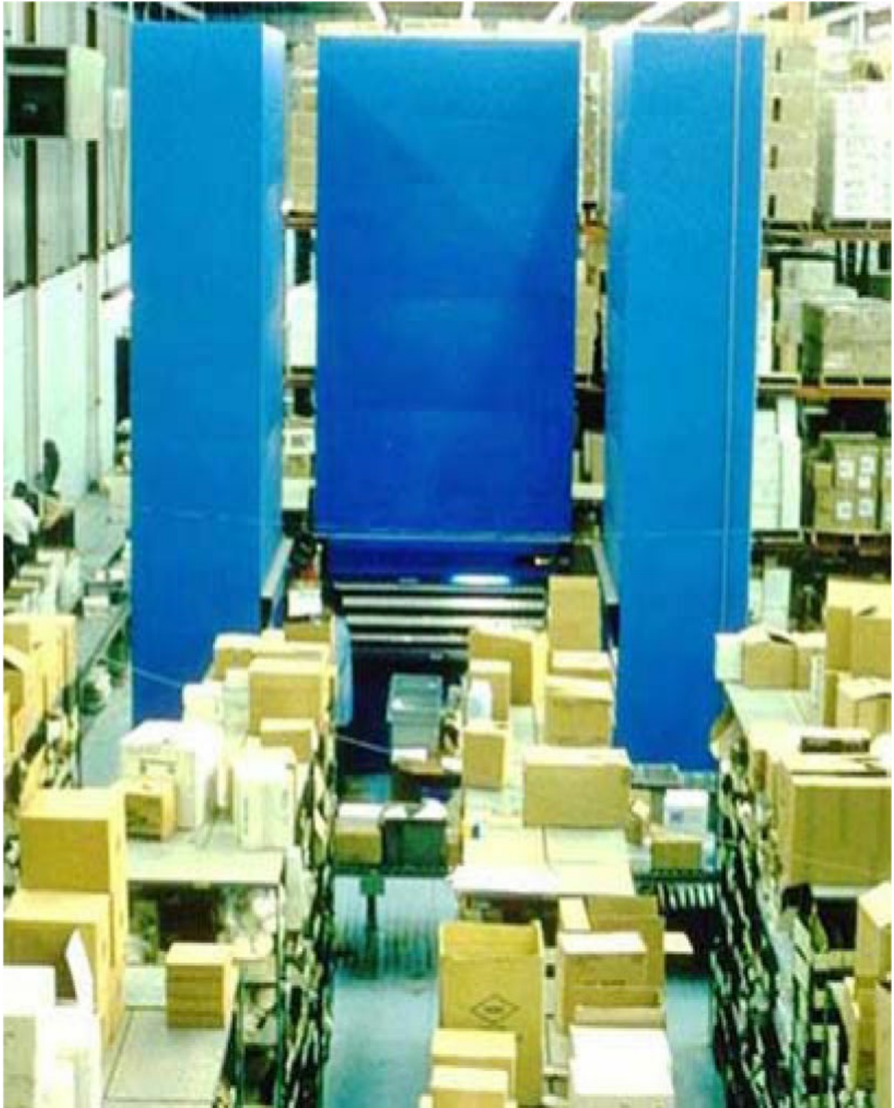
Figure 7.49 Vertical carousel installation at NASA.
